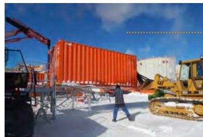
Installation du shelter HF
